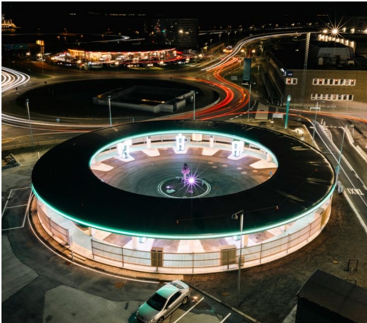
← The new charging station with 16 superchargers is easily accessible, located at one of the main roundabouts.
